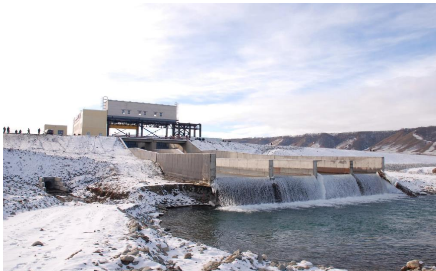
Fig.3 Small hydroelectric power station on the Bolshoy Zelenchuk river (the Karachay-Cherkess Republic)
