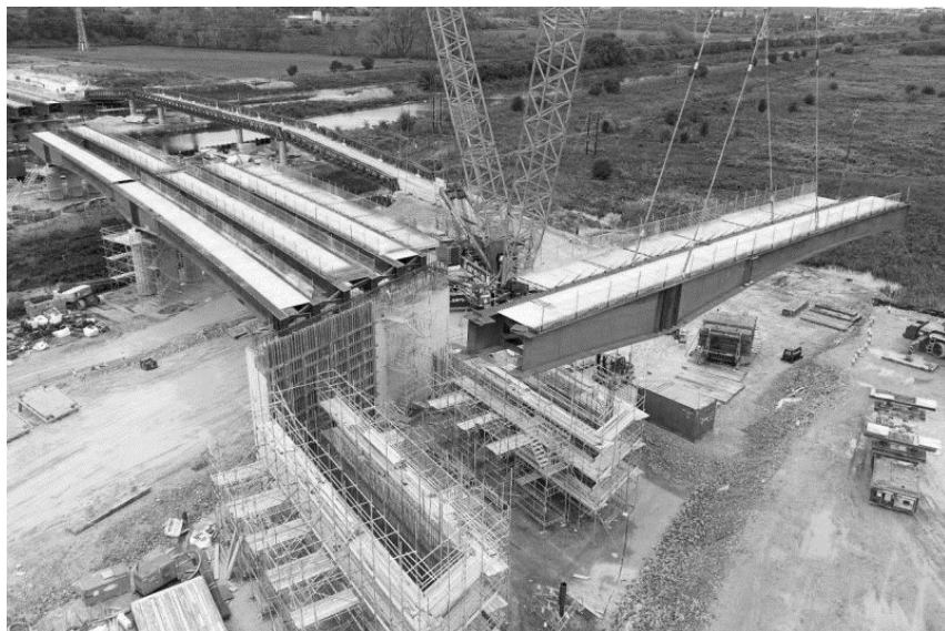
Рисунок 6. River Witham Bridge, Lincolnshire
