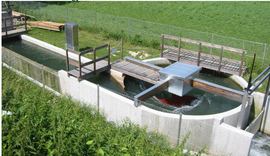
Fig.2. Micro-hydroelectric power station
