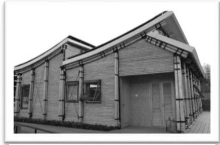
Fig.2. Bamboo for housing construction
